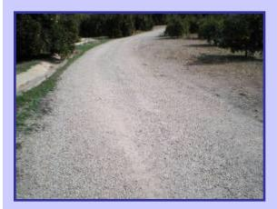
Gravel can be spread on roads to eliminate dust and retain sediment. However, this can be a relatively expensive project for an orchard.
