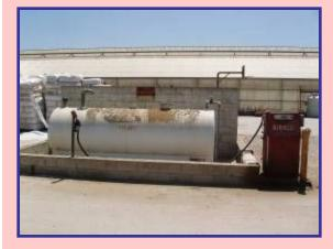
Fuel tanks should be located where they will not leak into groundwater or surface water.
