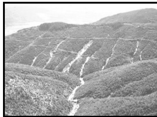
Figure 6. Road-induced debris flows in northwest Washington state, USA. The debris flows initiated in the colluvial hollows on the upper road were triggered by road runoff, and these triggered the failures at the road-stream crossings on the lower road. This sequence has been defined as a “disturbance cascade” (Wemple et al., 2001). The road was built prior to the implementation of best management practices and large fill volumes were placed within colluvial hollow and inner gorge landforms (WA DNR, 1983).
