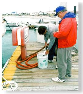
A sewage pumpout station being checked for efficiency. Waste pumped out from boats goes into the local sewage treatment system.
