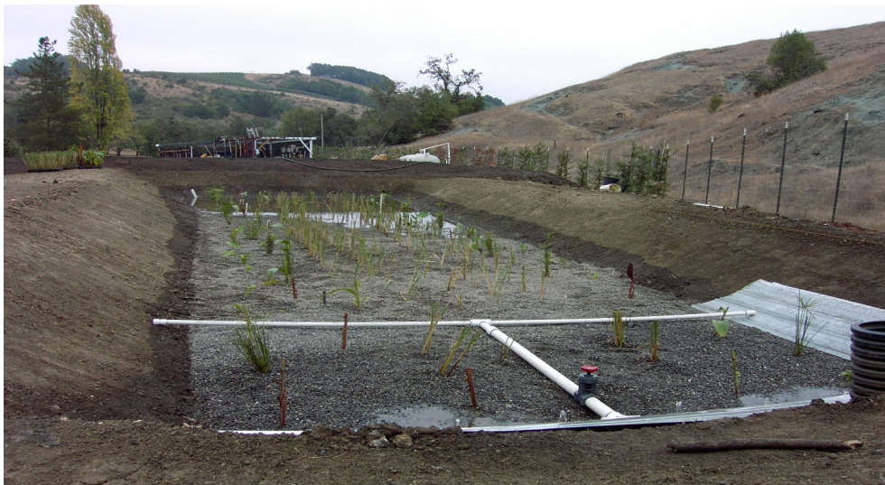
Figure 1: Newly constructed wetland for primary treatment of winery wastewater
