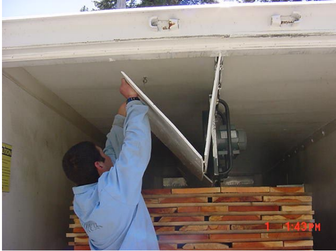
Figure 13. Lowering the Fan Baffles
