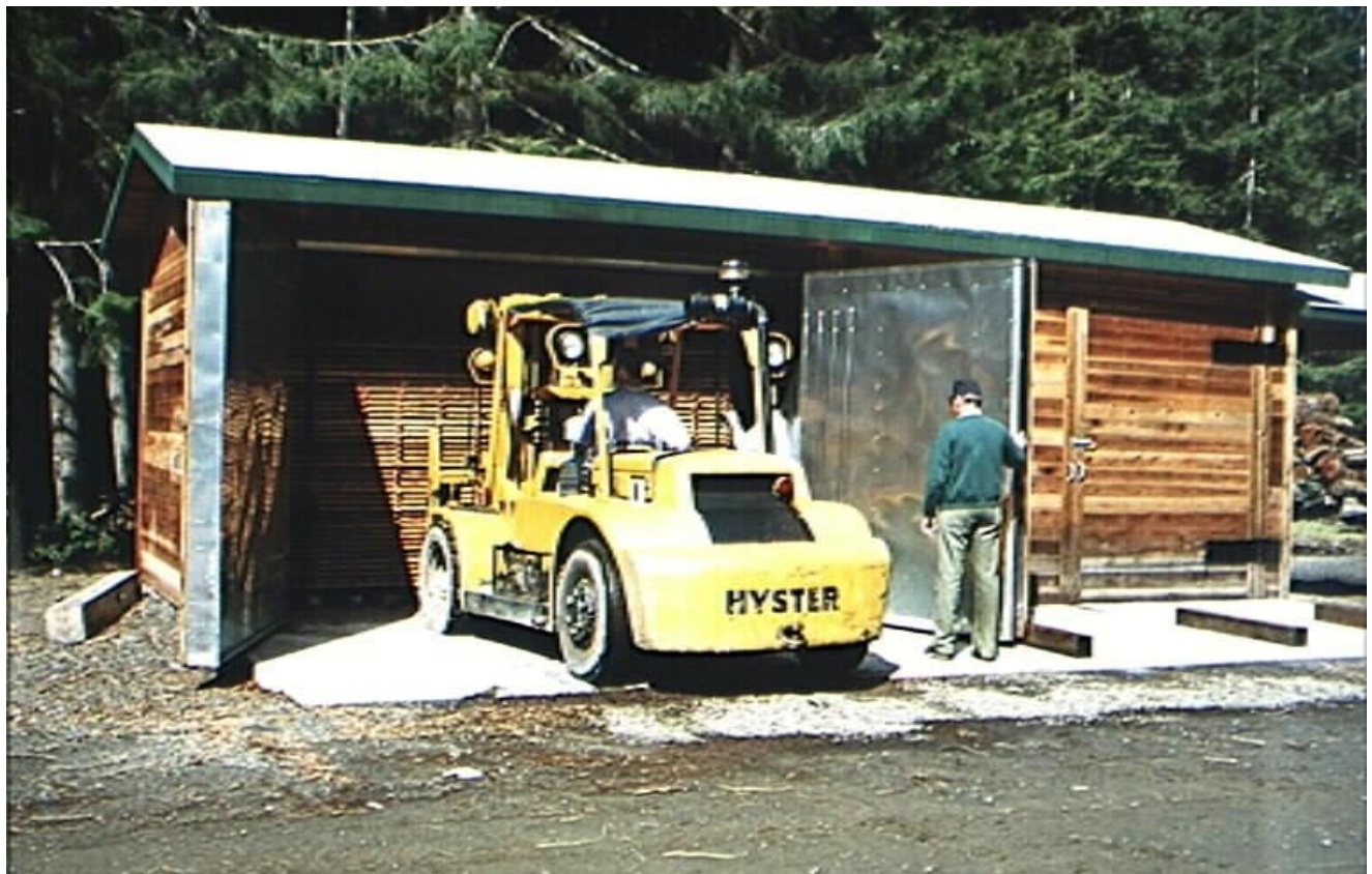
Figure 3. Two side-by-side forklift-loaded package lumber dry kilns. Each kiln houses a Nyle L200 Dehumidification unit and is designed for two units of 12 ft long lumber, one on top of the other (4,000 BF capacity each).
