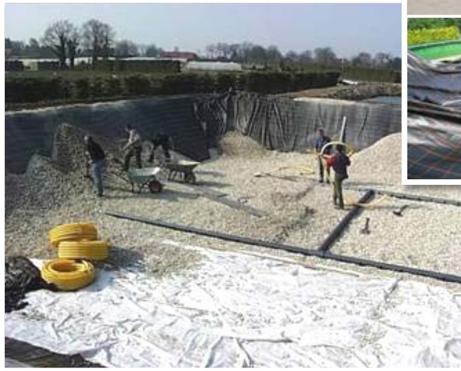
Underdrain system (lowest level)
